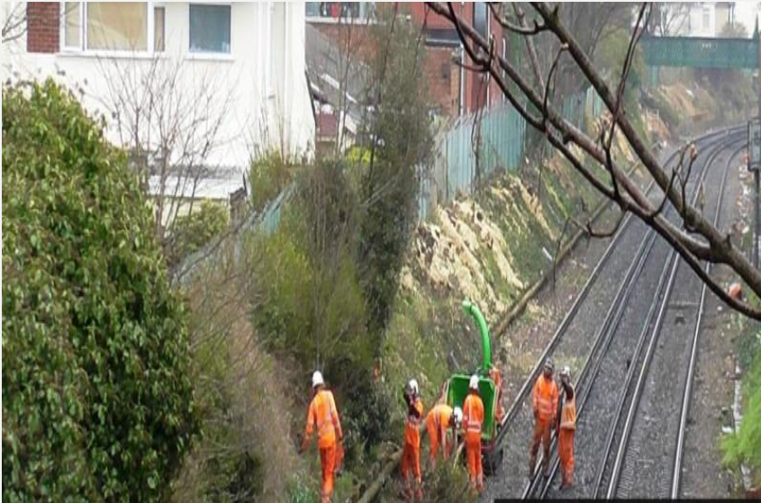
Clearance of trees on track embankment
